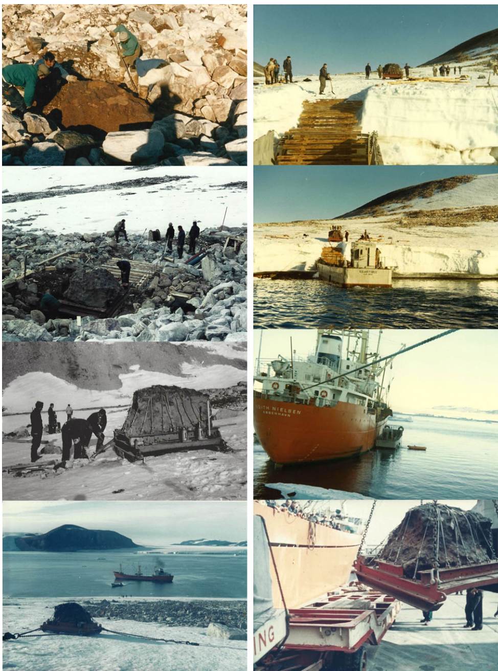
Fig. 4. Recovery of the Agpalilik meteorite, one of the Cape York meteorites. This is a time sequence running top to bottom left and then top to bottom right, the time period being 31st July 1963 to September 1967. The images show excavation with the help of Eskimos and dynamite, jacking up and building onto a sledge, hauling to the coastline, winching onto a U.S. Air Force landing craft, hoisting onto the M/S Edith Nielsen Danish supply ship, and placing on a truck for transfer to the Geological Museum of the University of Copenhagen.
