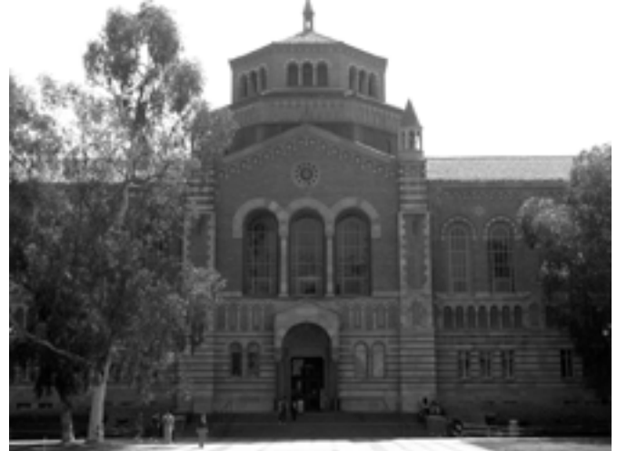
FIG. 2. Powell Library, as viewed from the front steps of contemporaneous Royce Hall. Powell Library's architecture was inspired by two structures from 12th century Italy. The octagonal tower is styled after part of the Complesso Monumentale di Santo Stefano in Bologna (in turn modeled after the 5th century tower of San Sepolcro in Jerusalem). The front entrance is modeled after the Basilica di San Zeno Maggiore in Verona.
